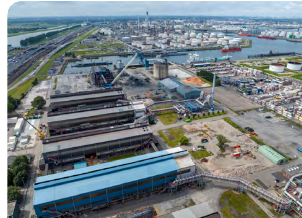
Demolition work of the Aluchemie factory in full swing (August 2023)
