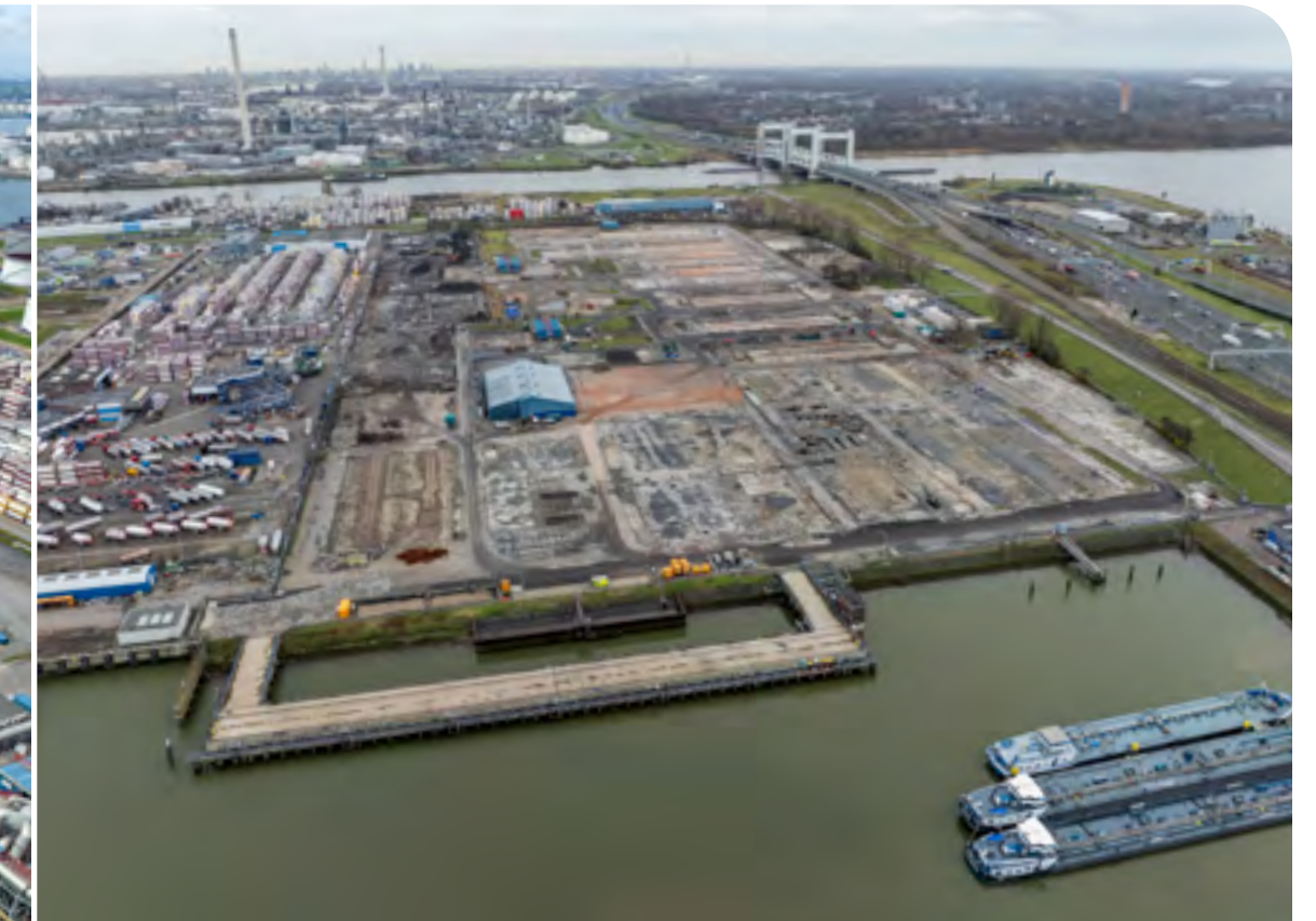
The site in December 2023, after most above-ground infrastructure has been demolished
